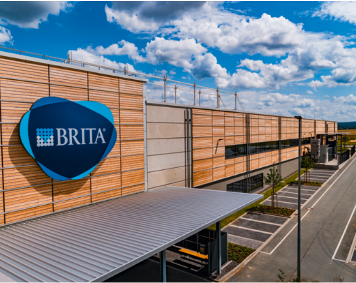
Groundbreaking: The energy-efficient new production site in Bad Camberg, Germany, is a timber hybrid building.
