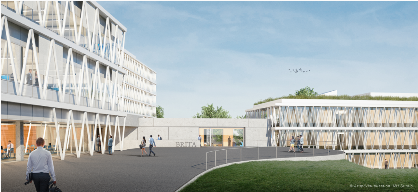
Sustainable and with a view to the future: A new office building will be constructed at the BRITA Campus in Taunusstein, Germany.
